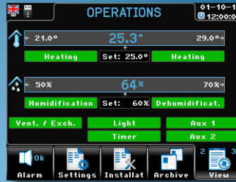
Viewing operating condition
